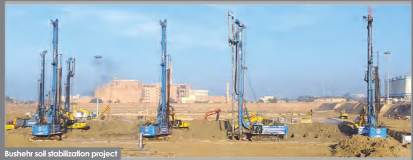
Bushehr soil stabilization project
