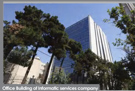
Office Building of Informatic services company
