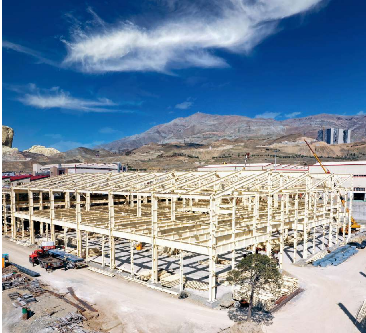
• Steel Structure for Southern Halls at Crouse Company Site No.3 | 11,000 tons
