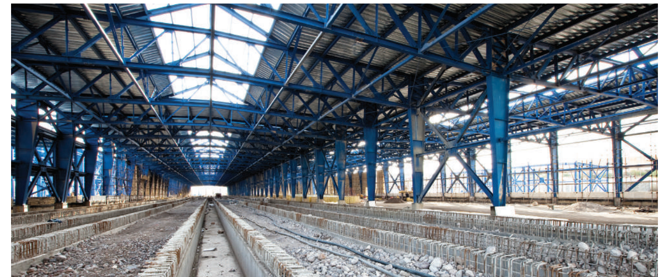
• Steel Structure for Industrial Sheds at Laleh Depot (Tabriz Metro) | 4,000 tons
