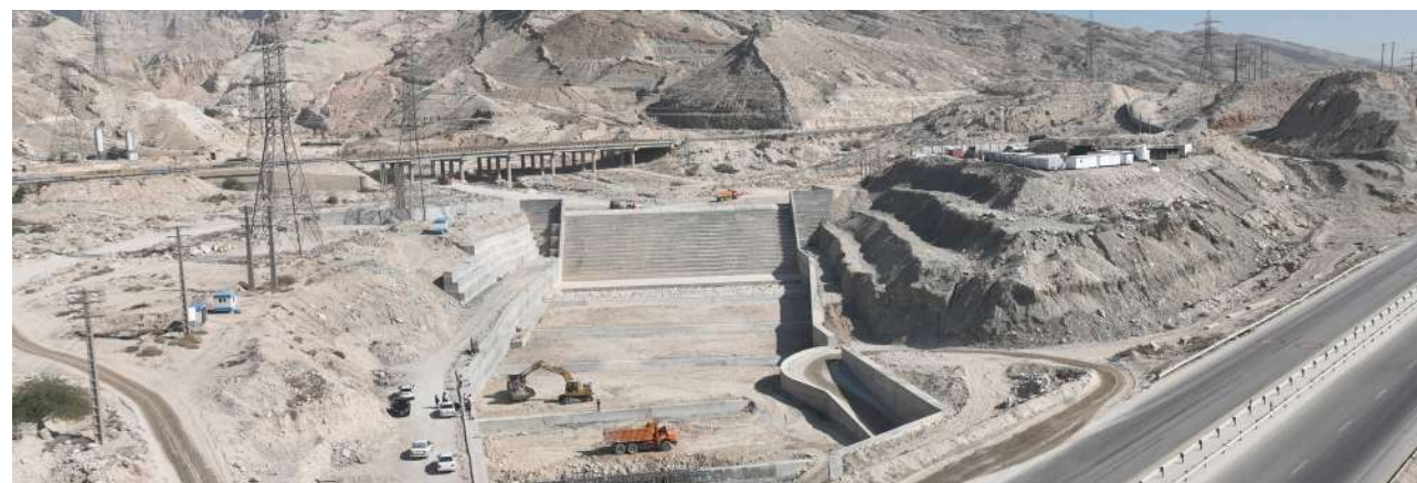
• Concrete Bed Stabilization Dam (Bedsill), Hanwies River
