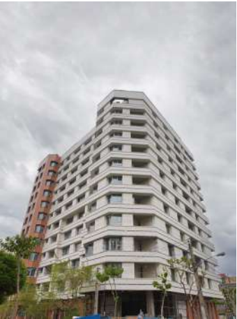
• 42-Unit Ajoudanieh Residential Complex
